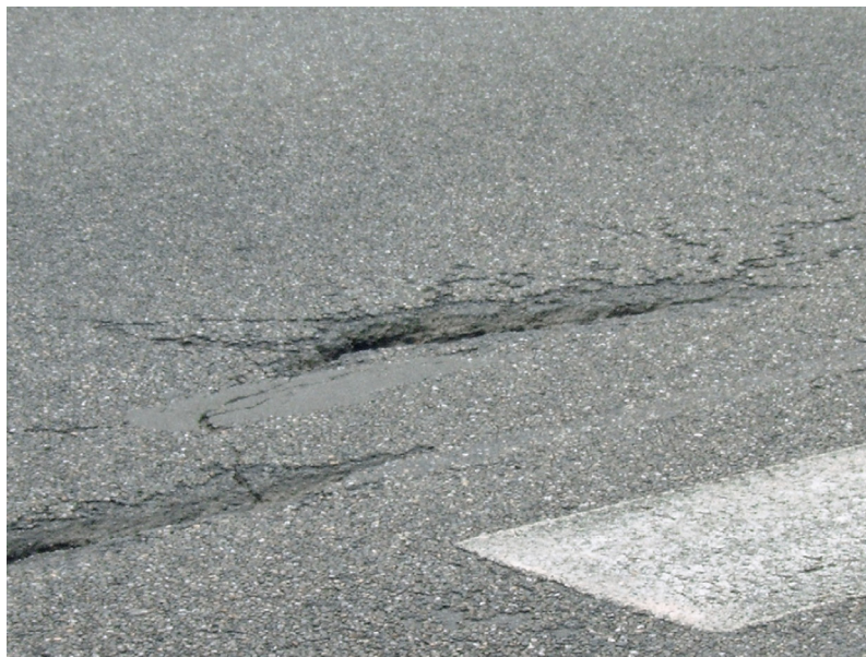
Picture 6: Potholes/fissures
