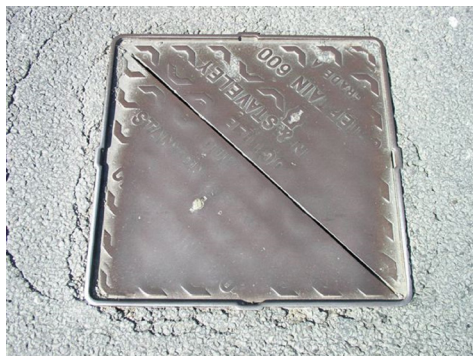
Figure 10 : Manhole cover before anti-skid treatment
