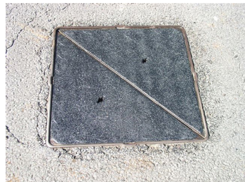
Figure 11 : Manhole cover after anti-skid treatment
