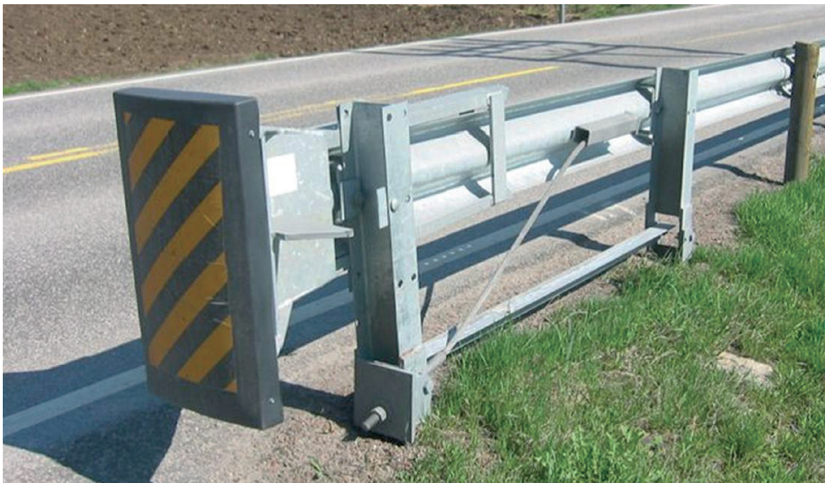
Figure 13 : Guardrail post as seen from the back of the barrier.
